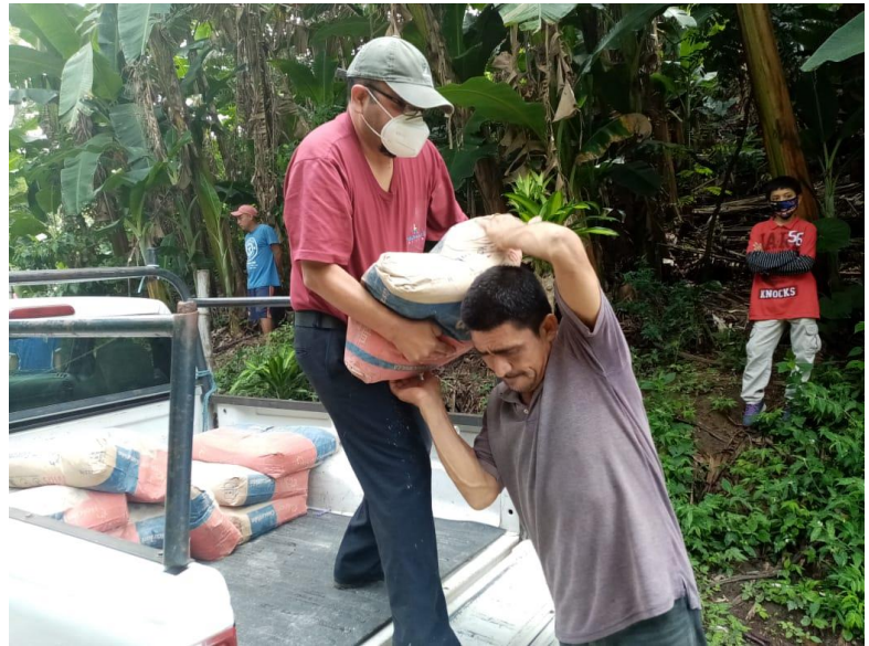
STARTING TO REPAIR THE DAMAGE
